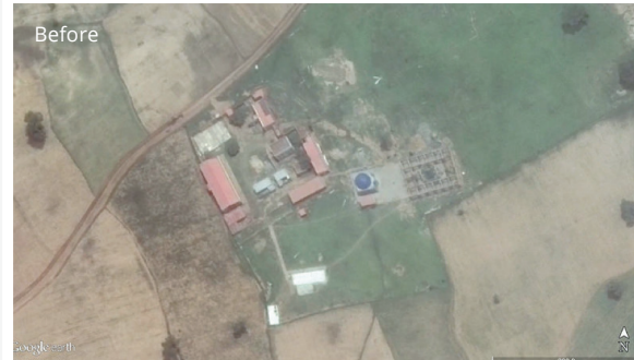
Example 1: Demolition of Mosque
